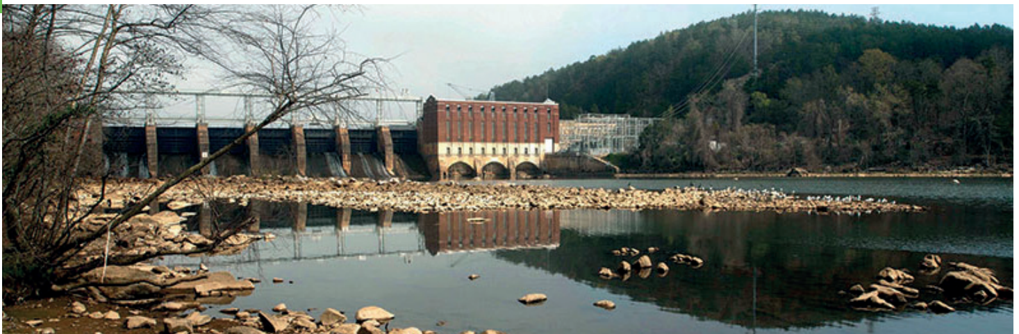
High Rock Lake Dam Yadkin River, Rowan County
